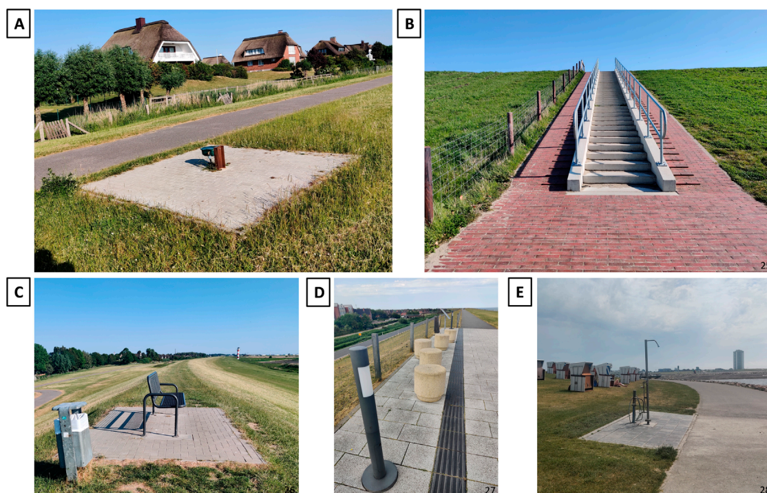
FIGURE 6 Exemplary photos of paving at transitions (©Ina Schulte 2023): (A) trough on landside, (B) stairways on landside, (C) bench on crest, (D) poles and objects on crest, (E) shower on seaside.
