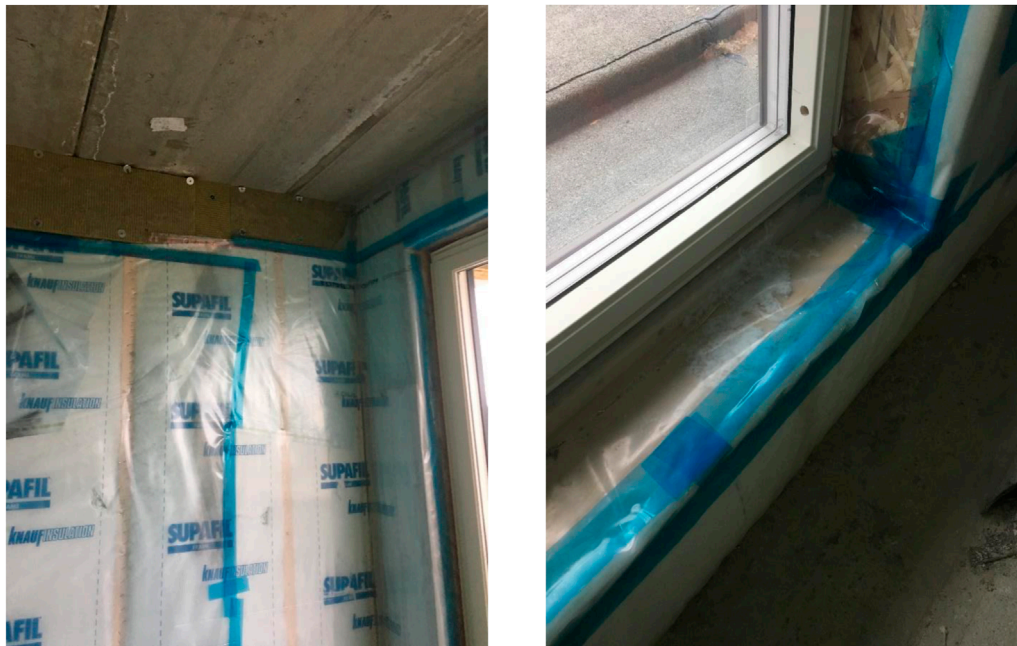
FIGURE 3 Adhesive tape is used to join sheets of vapor barrier membrane, and to connect the membrane to the timber frame (Photo: Geving S., SINTEF Community).
