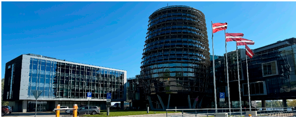
FIGURE 4 The office building complex of the case study (Source: own).
