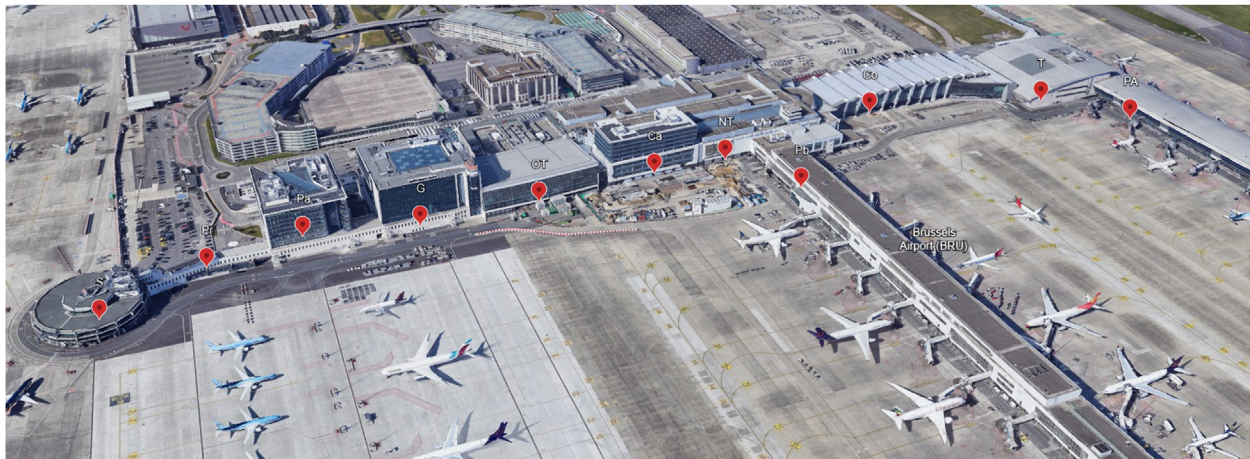
FIGURE 1 Core terminal buildings included in the analysis. Map data from: Google; data SIO, NOAA, U.S. Navy, NGA, GEBCO; IBCAO. Imagery from the dates 14/12/2015–18/07/2022.
