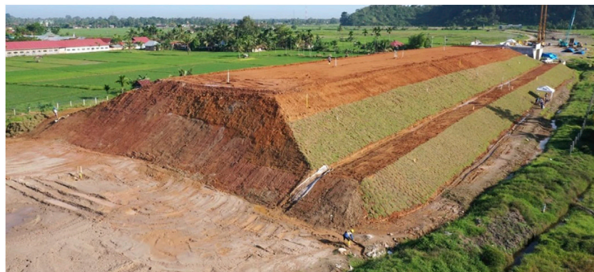
FIGURE 8 Trial embankment at the maximum height.
