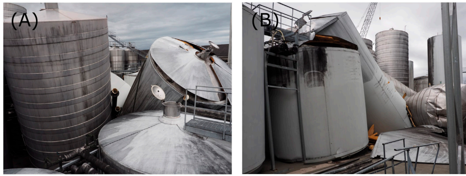
FIGURE 9 (A, B) Global collapse of slender tanks causing a cascade effect on neighbour tanks.
