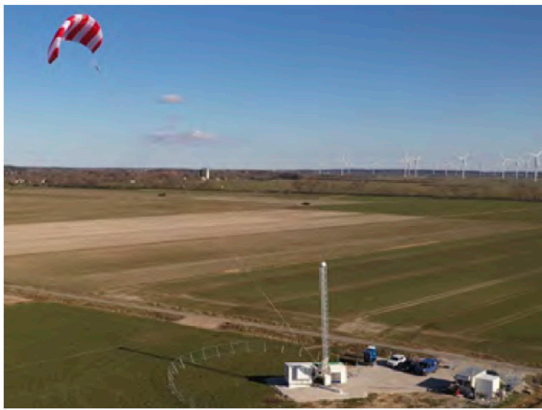
FIGURE 1 AWE Ground-Gen systems (SkySails, no date).
