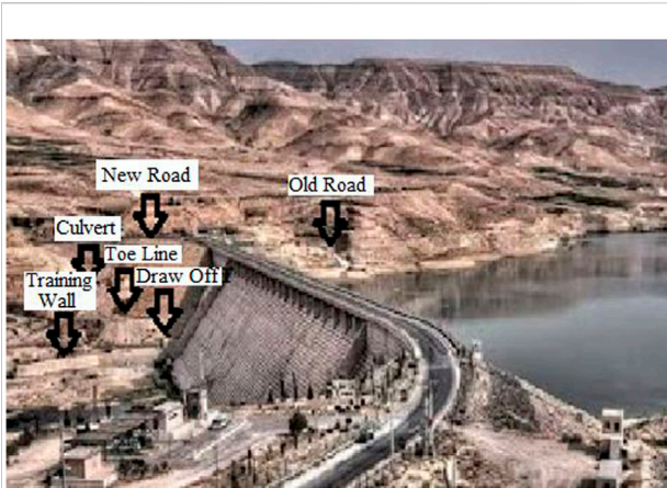
FIGURE 5 Location of various dam appurtenances.
