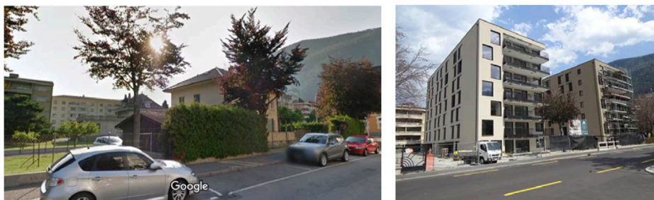
FIGURE 13 Martigny, two low-rise URM buildings demolished and replaced by a group of three identical mid-rise RC buildings (only two of them are visible on the right picture).
