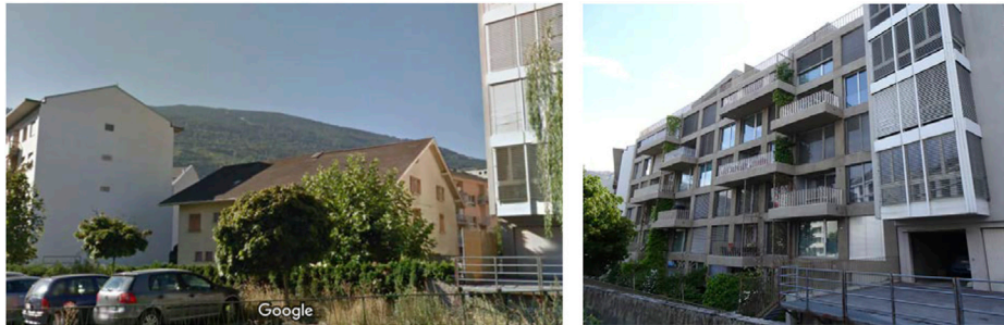
FIGURE 8 Sion, low-rise URM building demolished and replaced by a mid-rise RC building inserted between two adjacent buildings.
