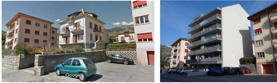
FIGURE 7 Sion, low-rise URM building demolished and replaced by a mid-rise RC building.
