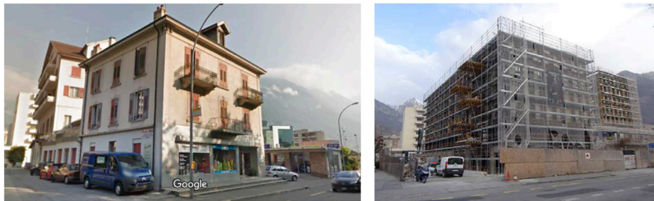
FIGURE 12 Martigny, two URM buildings demolished and replaced by a complex of two large high-rise RC buildings connected at their base by shared parking areas.
