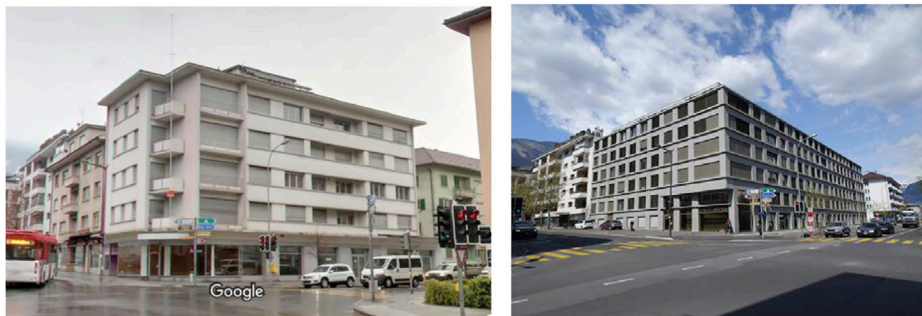
FIGURE 9 Sion, three URM and RC buildings demolished and replaced by a single large mid-rise RC building with a "U" plan shape.
