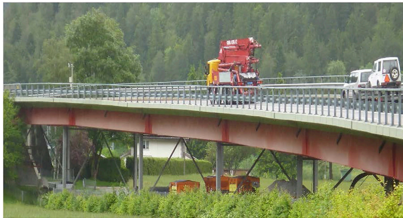
FIGURE 1 The composite steel-concrete bridge case study in Switzerland.
