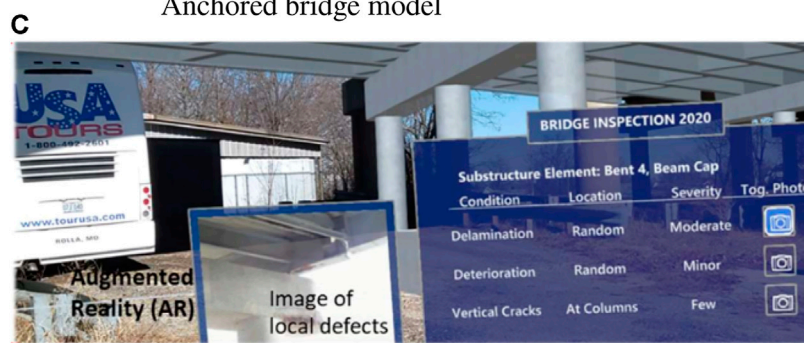
Hand-free bridge inspection enabled by AR interface
