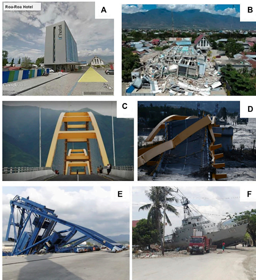
FIGURE 6 | Damage induced by the Palu Earthquake and Tsunami: Roa-Roa Hotel in Palu, built in 2013, (A) before the earthquake and (B) after the earthquake, steel double arch Palu Bridge IV over the mouth of the Palu River (C) before the earthquake and (D) after the earthquake and tsunami; (E) collapse of gantry crane in the Port of Pantoloan due to earthquake shaking; (F) naval ship washed ashore at Watusampu Naval Base.
