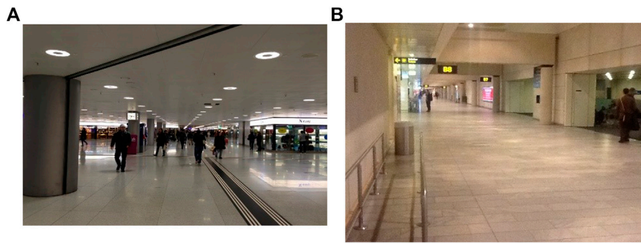
FIGURE 1 | The fireproof non-load-bearing walls: (A) The screen structures in the trade center; (B) The screen structures in the airport terminal.
