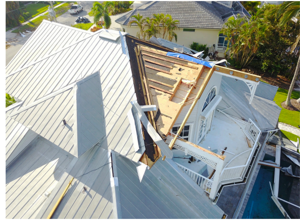
FIGURE 7 | UAVs with high-resolution cameras are well-suited capture perishable data (e.g., roof cover damage, debris field), and provide complementary datasets for ground-based damage surveys. The aerial perspective of UAVs reveals structural damage that is hidden from the view of ground-based damage surveyors. Photograph by Kwasi Oerry was acquired under sponsorship from the Florida Building Commission.
