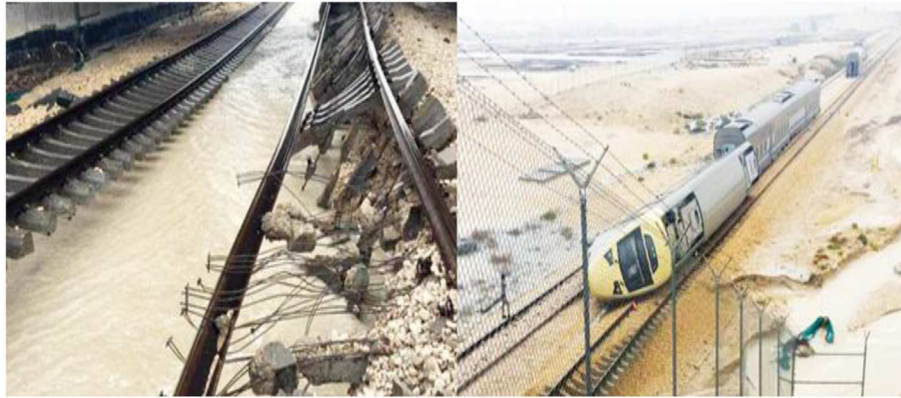
FIGURE 5 | Railway track inundated by water (left) and a train derailment near Dammam (right). Source: (Arabnews, 2017a).
