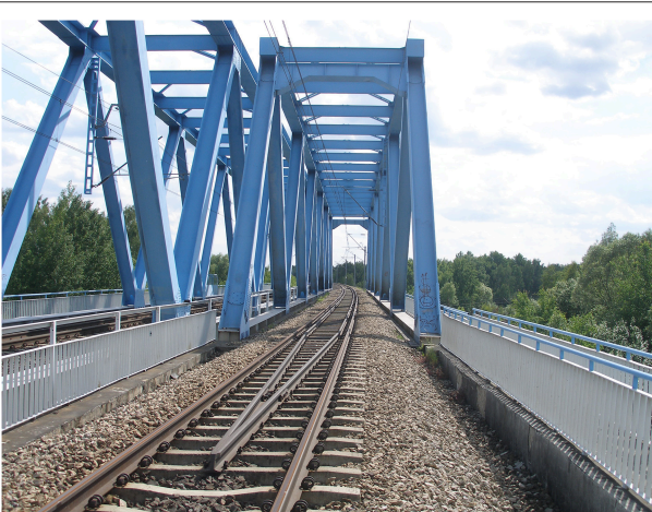
FIGURE 7 | View of the bridge from the railroad level-visible curved railway track; from Olaszek (2015) permission was granted by The Committee on Civil Engineering and Hydroengineering of the Polish Academy of Sciences.
