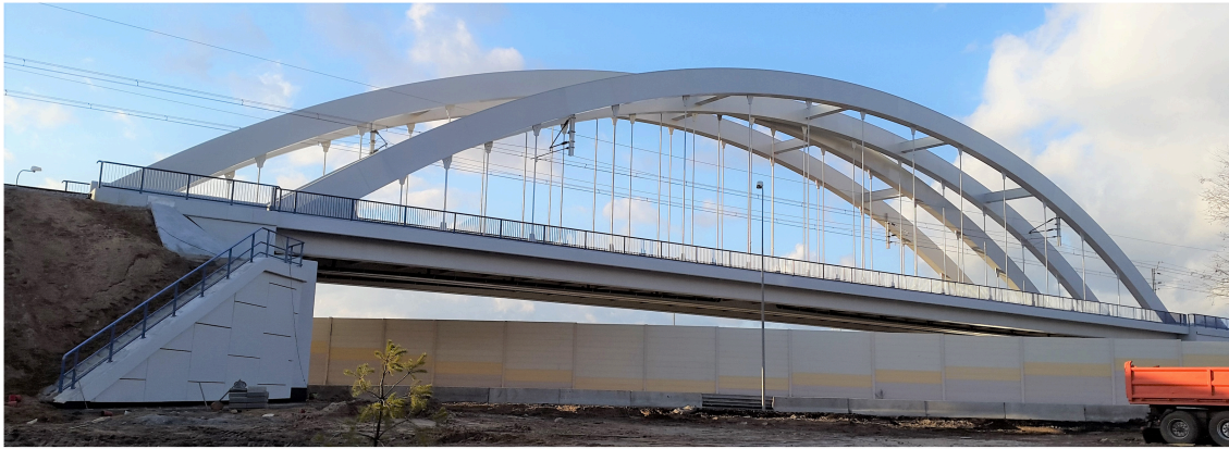
FIGURE 11 | Lateral view of the second railway bridge.
