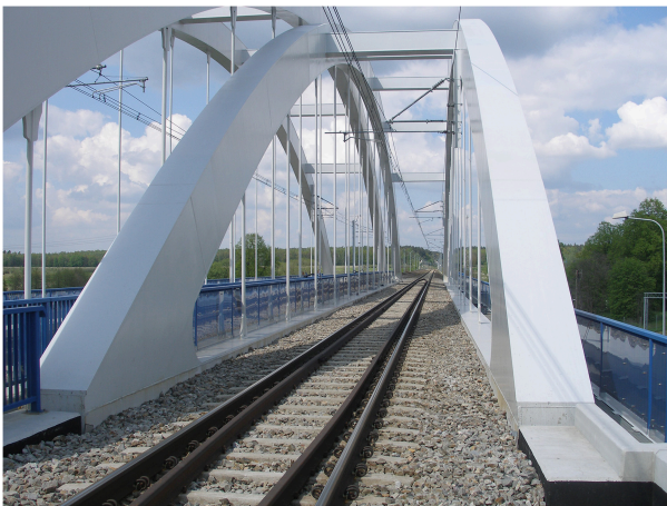
FIGURE 12 | View of the bridge from the railroad level—visible hangers made from steel bars.
