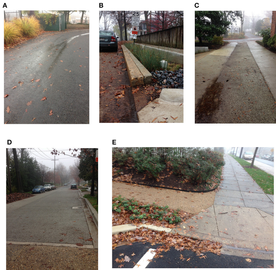
FIGURE 3 | Site Photographs of BMPs treating the sewershed's public ROWs. (A) Permeable asphalt: surface runoff is visible, indicating lower than expected infiltration performance. (B) Bioswale with a flush curb cut extending beyond the ROW into adjacent grass strip. (C) Permeable concrete installed in the center of a reverse crowned alley. (D) Permeable concrete spanning the full width of the ROW. (E) Foreground shows permeable rubber sidewalk adjacent to bioswale. Permeable pavers in parking lane are visible in the background.
