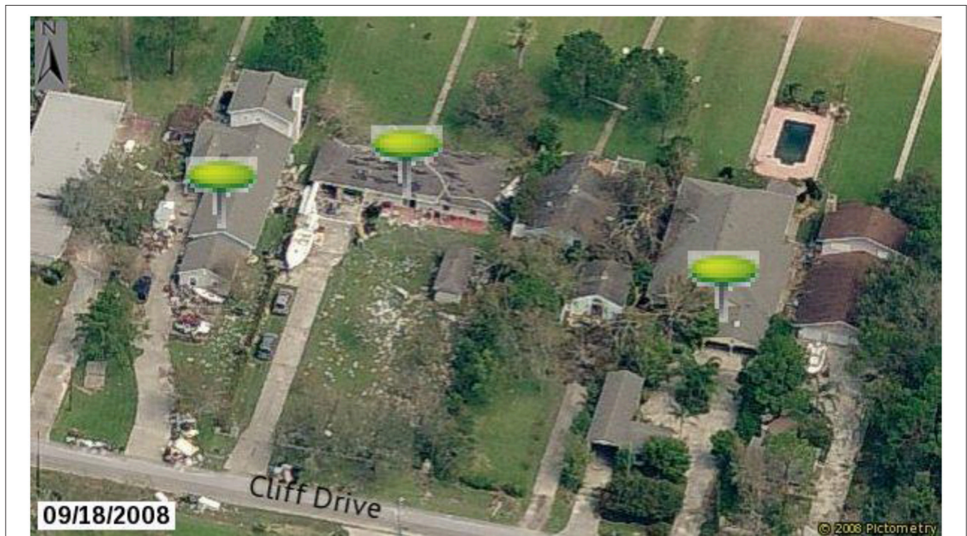
FIGURE 2 | Example oblique Pictometry image shows the condition of roofs and walls for one elevation. Data from additional viewpoint angles can be used to assess damage to the other three elevations of each building. Image resolution and quality reduced for publication. Pin icons denote houses that were included in the dataset. Varying colors of pins were for internal organization purposes only. Image courtesy of Eagleview Technologies, Inc.
