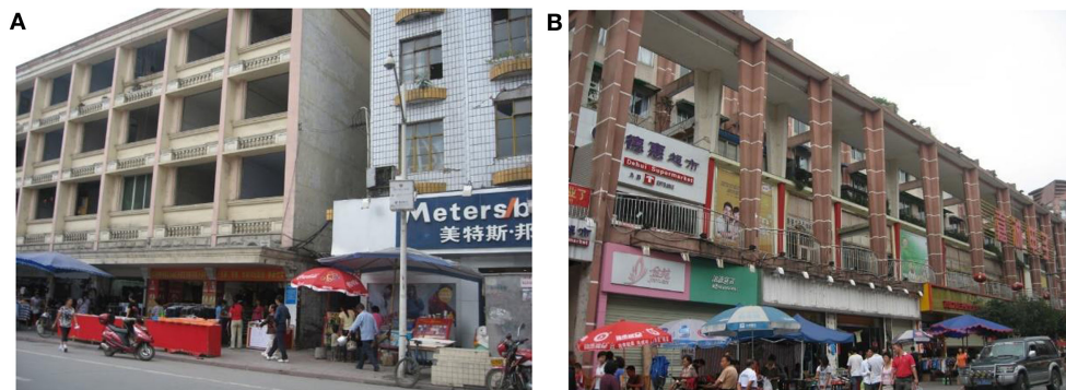
FIGURE 3 | Examples of existing buildings. (A) Typical reinforced concrete building and (B) multistory building with stores.
