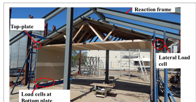
FIGURE 9 | Full-scale tests on house cross-section.
