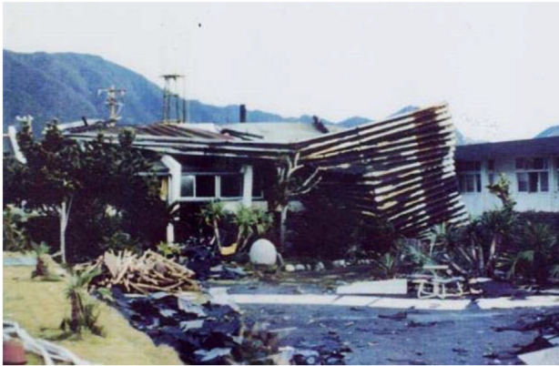
FIGURE 2 | Debris impacts, Typhoon 7513 at Hachijo Island, Tokyo, Japan.
