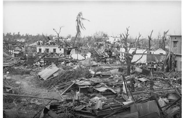
FIGURE 3 | Tornado damage in Manikganj, Bangladesh, April 1989. 1
