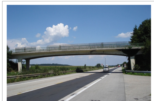
FIGURE 8 | S101 Bridge [Vienna Consulting Engineers (VCE), 2009].
