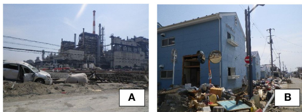
FIGURE 6 | Damage in Ishinomaki City: (A) photograph of an industrial area and (B) photograph of a residential area (photograph date: 15/4/2011).
