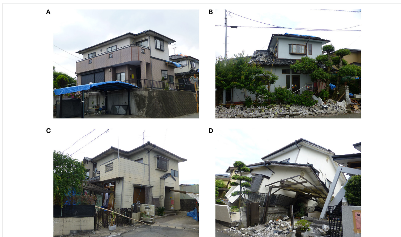
FIGURE 14 | Examples of damaged and collapsed timber buildings in Mashiki Town: (A) slight damage, (B) moderate damage, (C) heavy damage, and (D) collapse.
