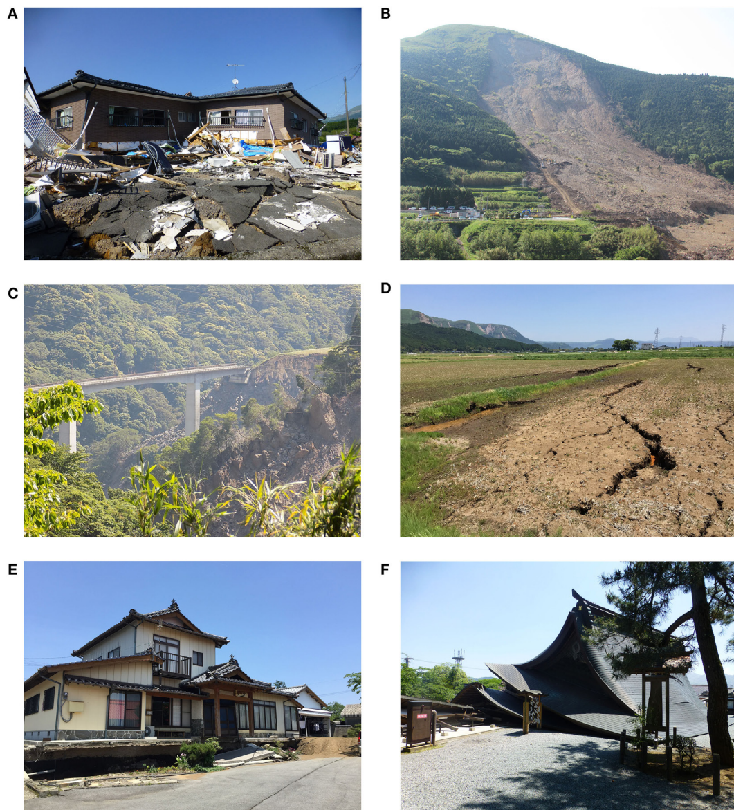
FIGURE 17 | (A) Collapsed timber building in the Kurokawa district of Minami Aso Village (Location 11 in Region 3). (B) Route 57 blockage due to the landslide near Aso bridge (location 11 in Region 3). (C) Damage to Choyo bridge (location 11 in Region 3). (D) Ground cracks near the Akamizu railway station (location 12 in region 3). (E) Ground settlement over a timber house (location 13 in region 3). (F) Collapse of Aso Shrine (location 14 in region 3).
