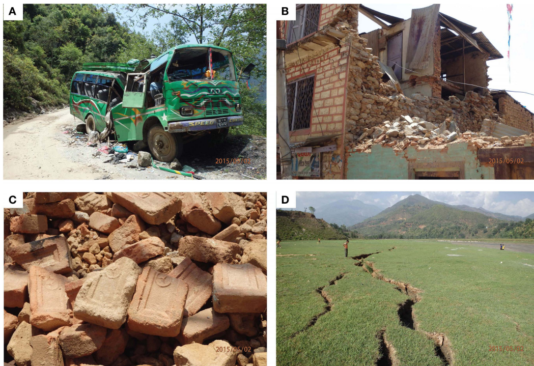
FIGURE 11 | Damage in Trishuli (see Figure 3). (A) Destroyed bus due to boulder fall. (B) Damaged brick masonry house in Battar. (C) Different types of bricks used in the damaged masonry house in Battar. (D) Ground fissures in the Trishuli dam reservoir.
