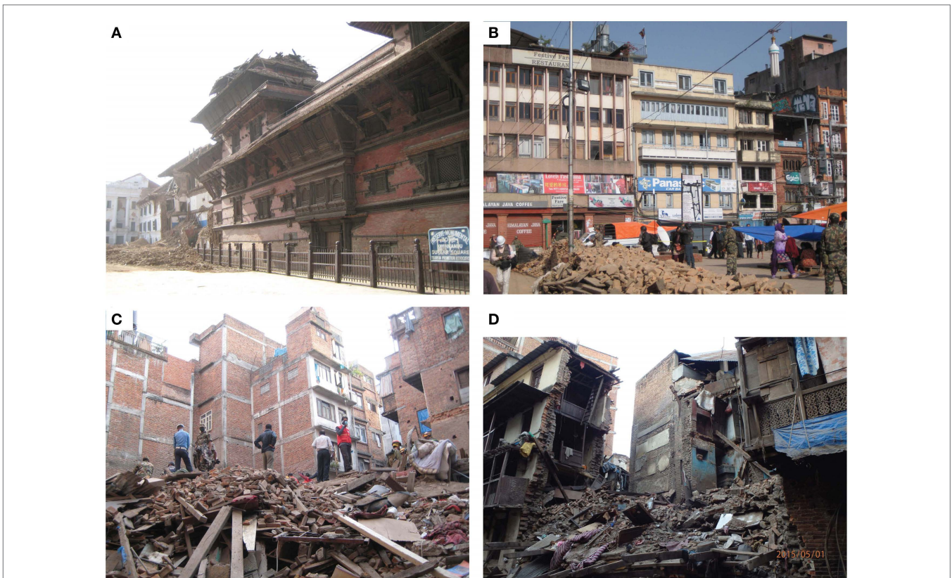
FIGURE 8 | Damage in Kathmandu (area 1 in Figure 4). (A) Collapse of the Basantapur Tower in the Kathmandu Durbar Square. (B) Undamaged buildings opposite of the Basantapur Tower in the Kathmandu Durbar Square. (C) Collapse of four 5- or 6-story old masonry buildings. (D) Collapse of a 4-story masonry building.
