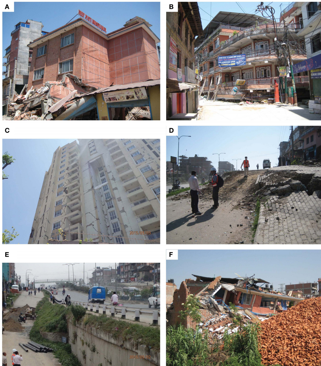
FIGURE 9 | Damage in Kathmandu (areas 2–5 in Figure 4). (A) Collapsed building along the Bishnumati River (alluvial soil deposit area; area 2 in Figure 4). (B) Collapsed building (soft story collapse) near the Bishnumati River (boundary between alluvial and Pleistocene soil deposit areas; area 2 in
