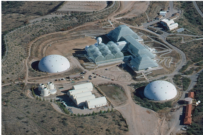
FIGURE 7 | The Biosphere 2 complex in Oracle, AZ was assembled in an open-construction configuration that permitted many more insect pests, plant diseases, and microbial communities than the closed-construction configurations of spacecraft, ISS modules (e.g., Figure 6 ), or future BLSS habitats. (Photo credit: A. C. Schuenger).
