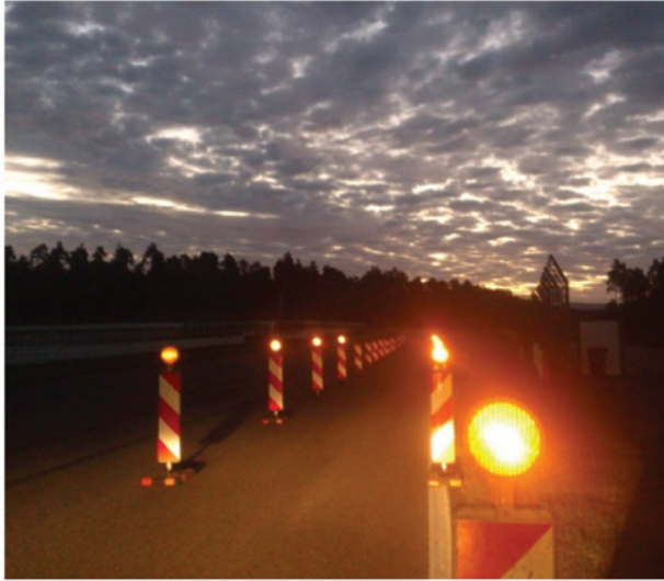
Figure 9: The built up construction zone at the Hockenheimring.
