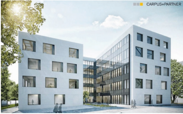
The new I3-RCDPP research facility is a further addition to the Digital Photonic Production research campus. © Carpus + Partner, Aachen, Germany.
