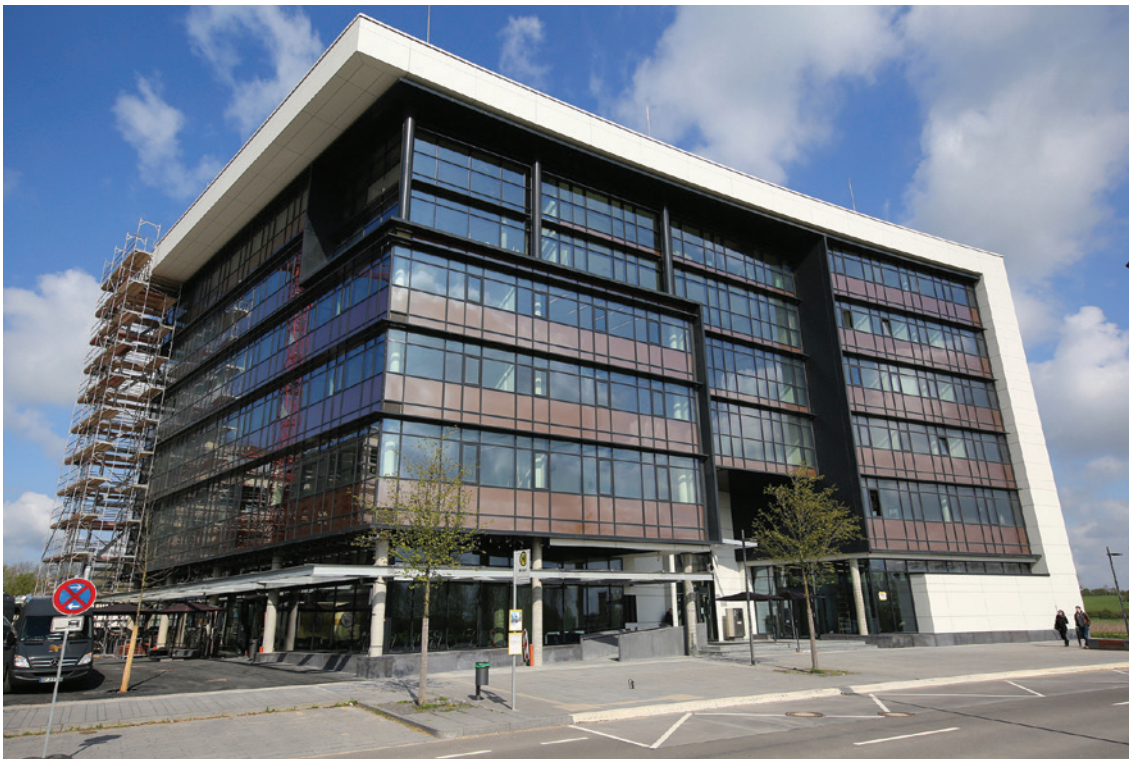
The first building of the Photonics Cluster on the RWTH Aachen Campus, now ready for its new tenants. The second building, due to be completed in 2018, is being built directly behind the first (Copyright: Fraunhofer ILT, Aachen/Andreas Steindl).
