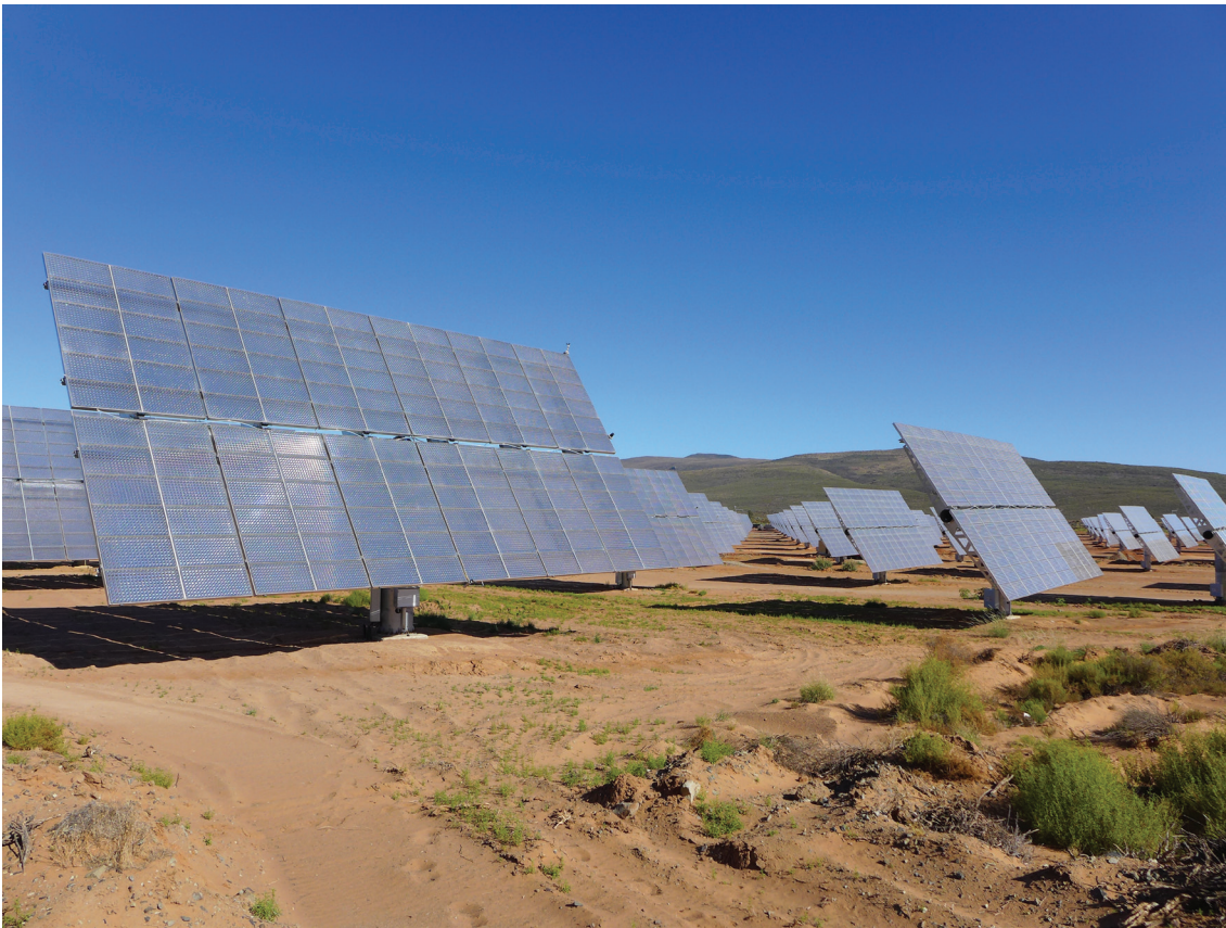
Figure 7 CPV power plant of Soitec Solar in Touwsrivier, South Africa. A capacity of 44 MW p is grid connected (Picture: © Soitec).
