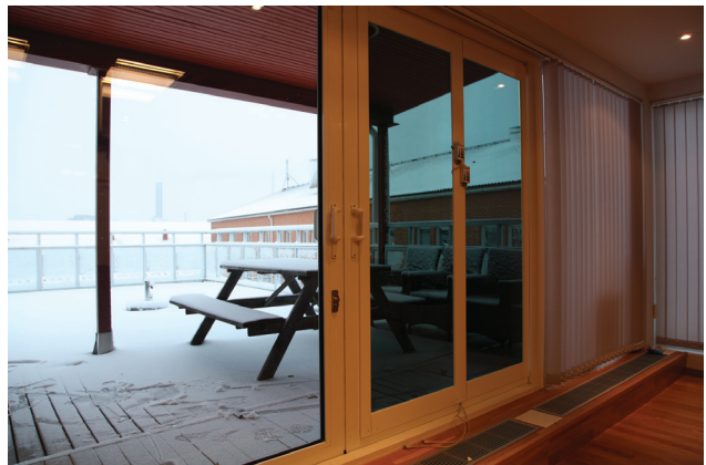
Figure 12 Part of an office equipped with electrochromic glazing, with one window being transparent and two windows in their dark state.
