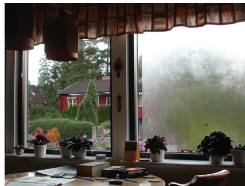
Figure 14 Photograph of a window on a private house in Uppsala, Sweden. Both parts of the window are triple glazed and have a center-of-glass thermal conductance as small as 0.65\text{ W/m}^2/\text{K} . The window is in a northeast-facing facade with an open view toward the sky. The left-hand part of the window has an outer glass with a self-cleaning and superhydrophilic \text{TiO}_2 -based coating, and the right-hand part employs standard uncoated glass. From Ref. [1].
