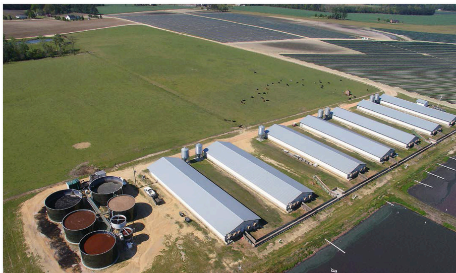
FIGURE 1 | Aerial picture of waste treatment system and barns. It treated all the manure flushed from seven barns with 735 pigs each. Existing lagoons are shown in the foreground.
