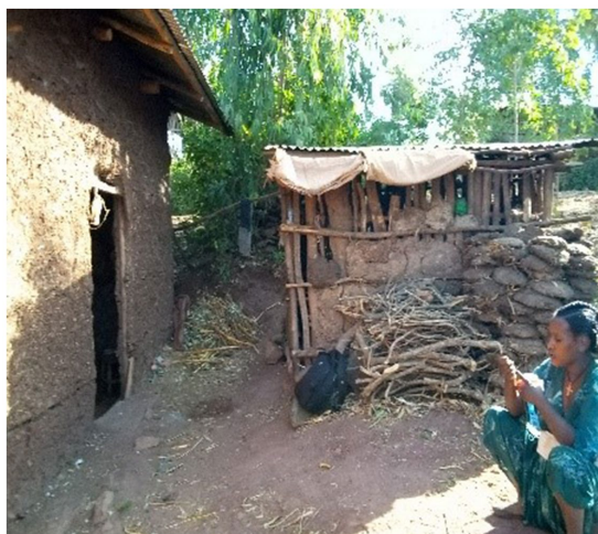
FIGURE 2 Small corrugated iron sheet roof kitchen near the main house.
