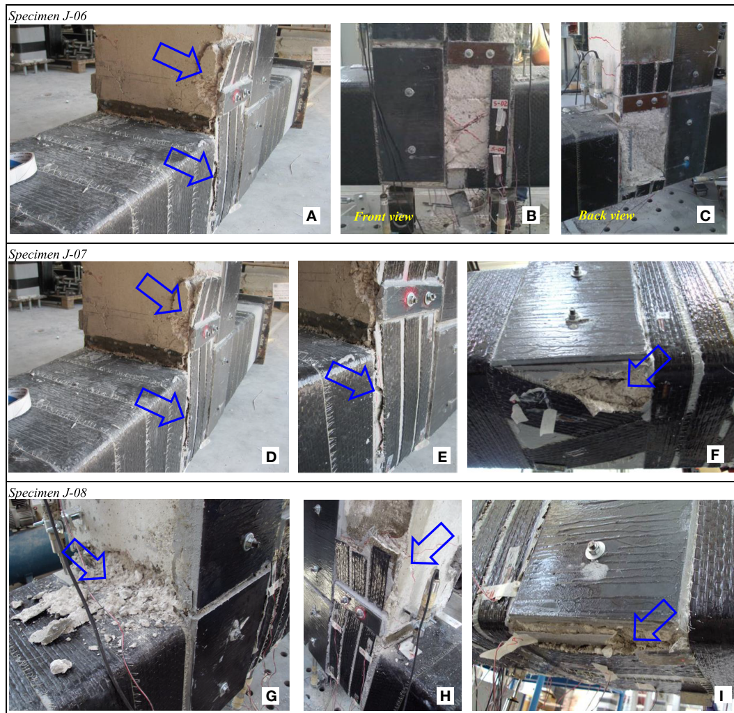
FIGURE 7 | Crack pattern and failure for CFRP strengthened specimens: J-06 (A-C); J-07 (D-F); J-08 (G-I).
