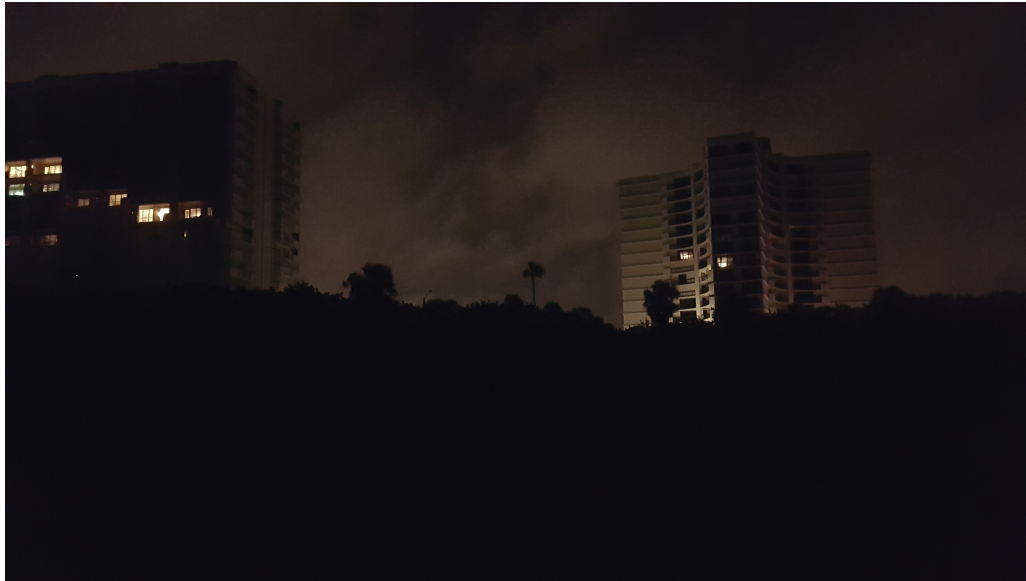
FIGURE 4 | Two condominiums in Boca Raton with sky glow and common urban lighting visible from the beach. Low clouds increase the reflection of lights from the adjacent city and sky glow. Sky glow is associated with hatchling disorientation.
