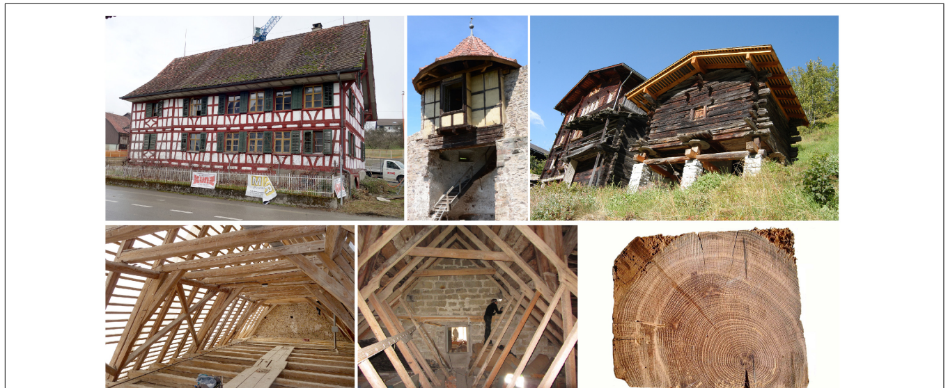
FIGURE 2 | Examples of type of buildings and material used to derive the felling dates from. Top: Half-timbered building in Sonterswil (Thurgau, Switzerland) from the 17th century. Tower of the town wall from Ribeauvillé (Alsace, France) from the 16th century. Log houses in the Lötschental Valley (Valais, Switzerland) from the 18th century. Below: Roof truss of the Chapelle Saint-Denis in Marmoutier (Alsace, France) from the 16th century. Roof truss from the church in Forshem, southwestern Sweden, with a nave from the 12th century and a chancel from the 13th century. Cross section of an oak beam from the Cathedral of Reims (France) from the 13th century.
