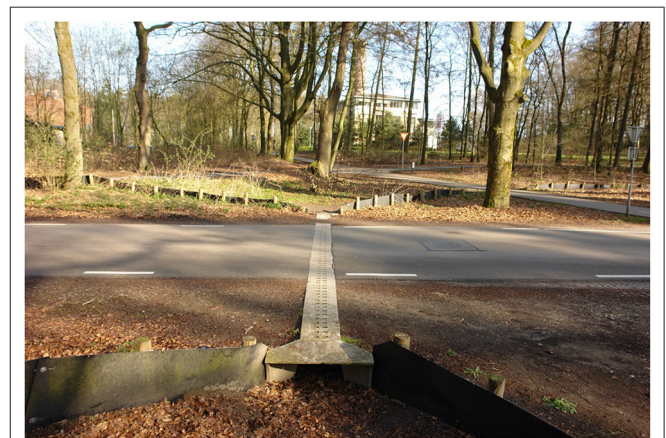
FIGURE 1 | Amphibian tunnel and drift fence at the study site. Photo: F. Ottburg.
