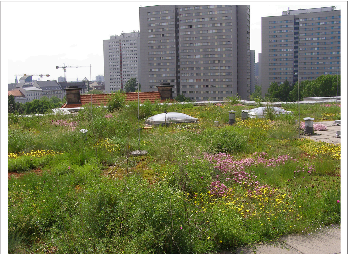
FIGURE 1 | A green roof comprised of shallow substrate and drought tolerant vegetation at the Berliner Wasserbetriebe in Berlin, Germany (Photo credit: Kelly Ksiazek-Mikenas).
