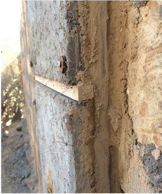
FIGURE 2 | Test wall using fiber cement panel and air gap in Bhuj.
