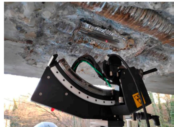
FIGURE 13 XRD tests execution on the bridge PTC beams.
