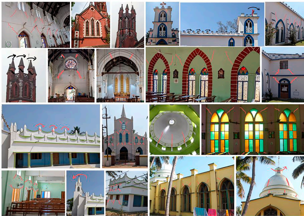
FIGURE 5 Possible collapse mechanisms in the analyzed churches.
