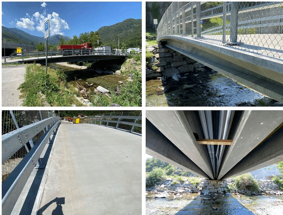
FIGURE 14 | Taverne bridge. (Photographs: E. Brühwiler).
