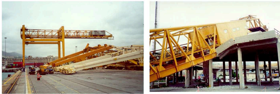
FIGURE 3 | Damage caused by a downburst in the seaport of Genova (August 31, 1994).
